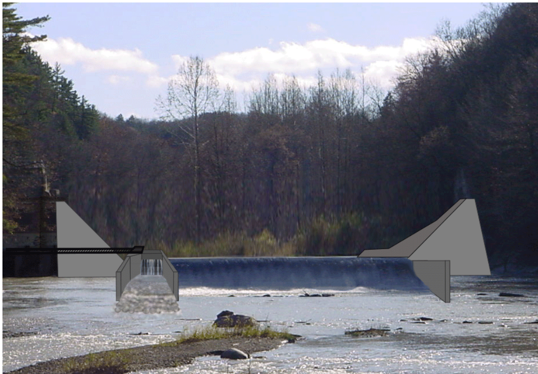
Figure 2. Springville Dam - Artist's rendering of completed fish passage ramp with sea lamprey barrier.
