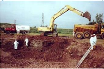
**Remediation of the Ashland 2 site was completed in September of 1999. Completed work entailed the excavation and disposal of 52,250 tons of soils containing radioactive residuals from the processing of uranium ores, backfilling and final restoration of the site.**
