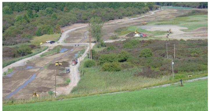
**This photograph shows the completed Rattlesnake Creek Project (completed in September 2005) with crews placing clean topsoil and seeding the site with indigenous plants. Nearly 33,300 tons of contaminated soils were excavated from the site and safely shipped out-of-state to a licensed disposal facility.**
