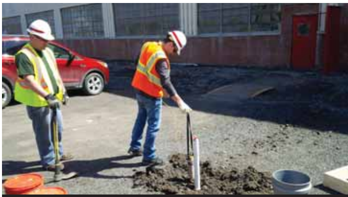
Monitoring well repairs at the Guterl Site
