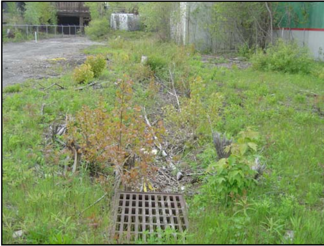
Photo 4 – View of a wet depressional area northwest of Bldg 35. The area is associated with a drainage swale.
