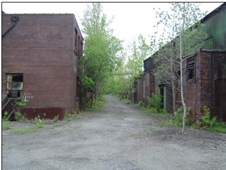
Photo 1 – View of the abandoned buildings and access ways within the parcel.
