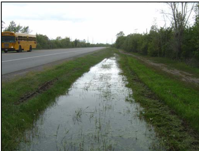
Photo 9 – View of the drainage swale located east of the Rt 93 bypass.
