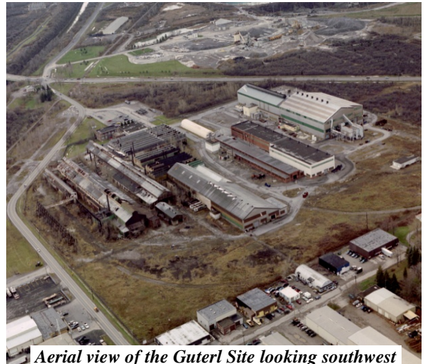
Aerial view of the Guterl Site looking southwest
