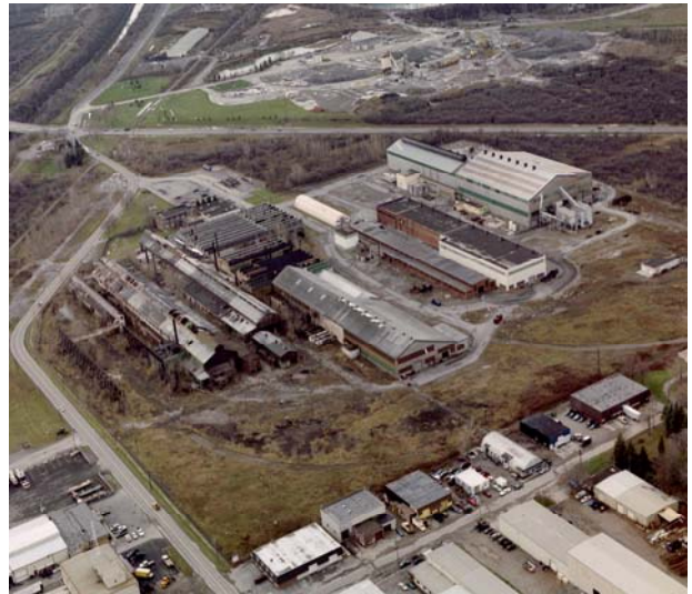
Aerial view looking southeast
