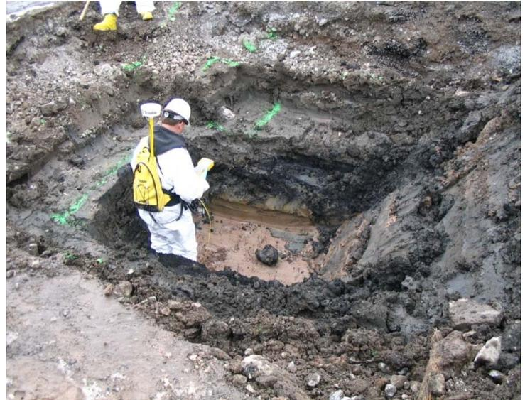
*Corps of Engineers Remediation of Contaminated Soil Lens (black) at Linde (circa 2010)*
