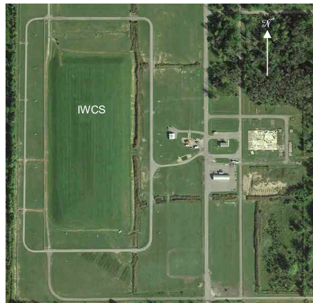
Figure 1: NFSS Interim Waste Containment Structure (IWCS)
