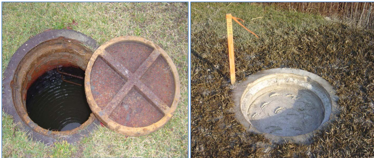
Photograph 5 - Manhole MH08 before and after plugging
