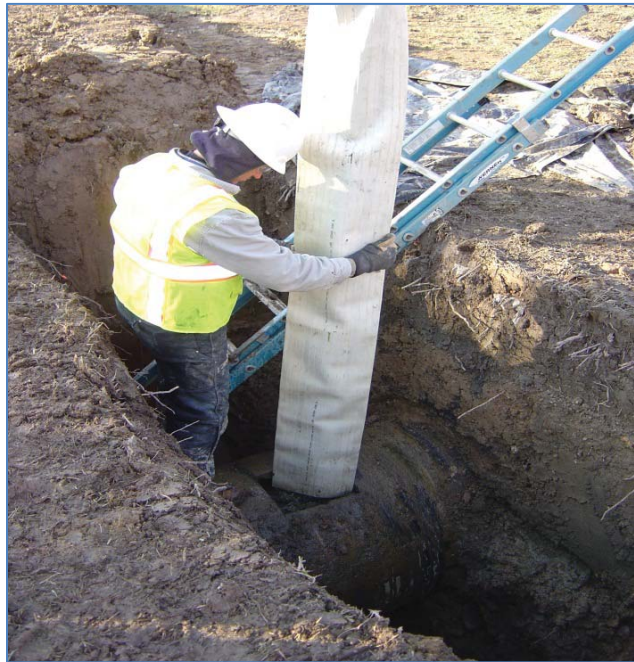
Photograph 4 - Concrete being pumped into 24-inch pipe in PE4
