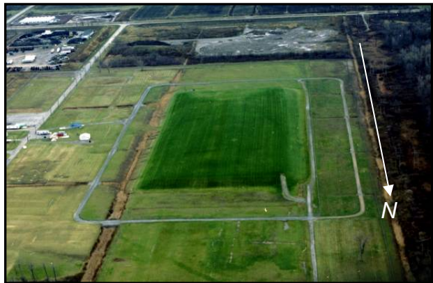
Figure 1: NFSS Interim Waste Containment Structure
