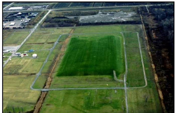
Figure 1: NFSS Interim Waste Containment Structure
