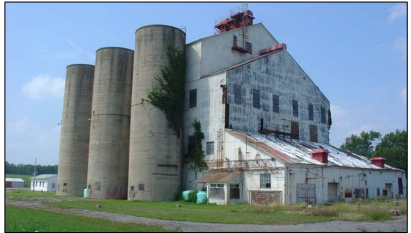
Building 401, Niagara Falls Storage Site, Lewiston, New York.
