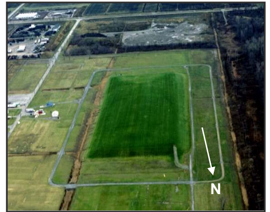
Figure 1: IWCS at the Niagara Falls Storage Site (looking south)
