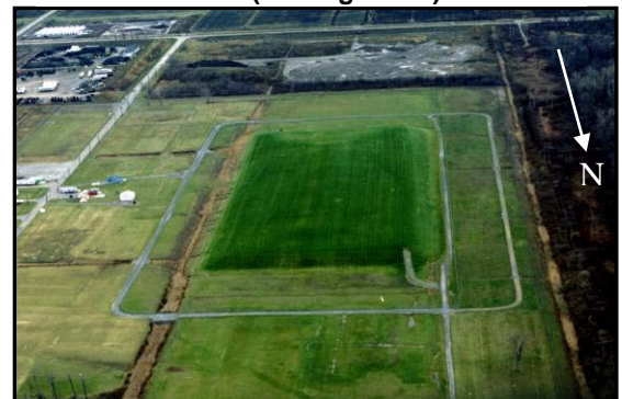
Interim Waste Containment Structure at the NFSS (looking south).
