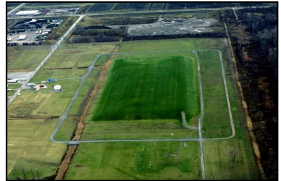
Figure 1: Interim Waste Containment Structure (IWCS) at the NFSS.
