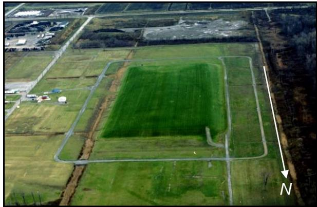
**Figure 1: NFSS Interim Waste Containment Structure**
