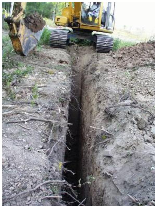
*Figure 4: Trench on VPG. This picture shows the start of the 65 foot-long, 12-foot deep trench began on May 22, 2002.*
