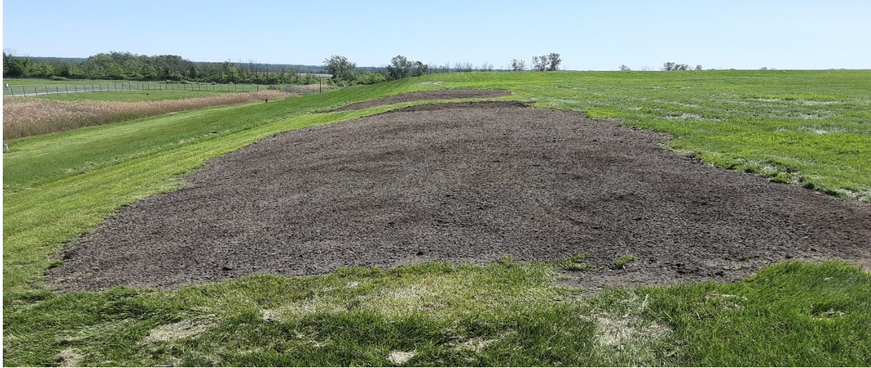
Figure 4: Topsoil enhancement on the IWCS
