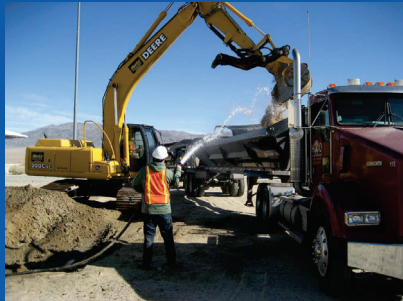
Dust control during excavation and loading
