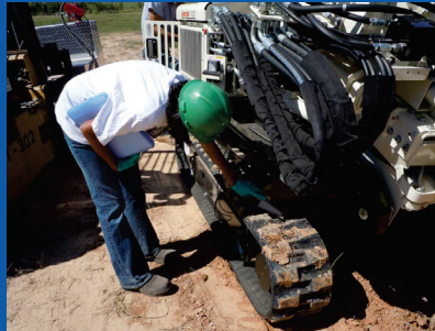
Scanning and decontamination of equipment and trucks exiting the contamination reduction zone
