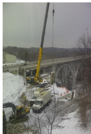
Demolition of Underpass Road and Bridges at NASA Glenn Research Center
