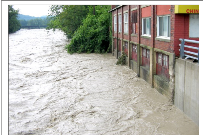
Figure 1: Flood water levels during 2009 flood event
