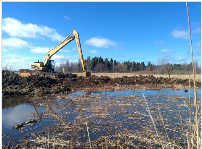
Channel clearing at Braddock Bay, April 2018
