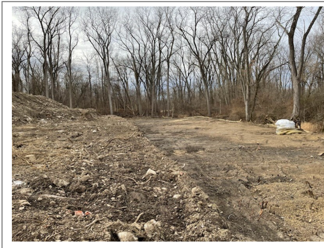
2A East Subsurface Debris Removal along Pipe Creek
