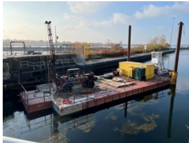
Geotech Work November 2022
