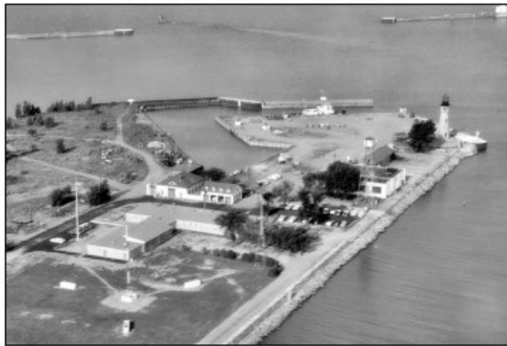
Figure 60. A 1962 aerial showing the removal of the concrete banquette and its replacement with rubble from the now demolished 1900 era banquette down the length of the mole (US Coast Guard).
