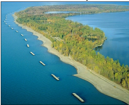
Aerial view of offshore breakwater project
