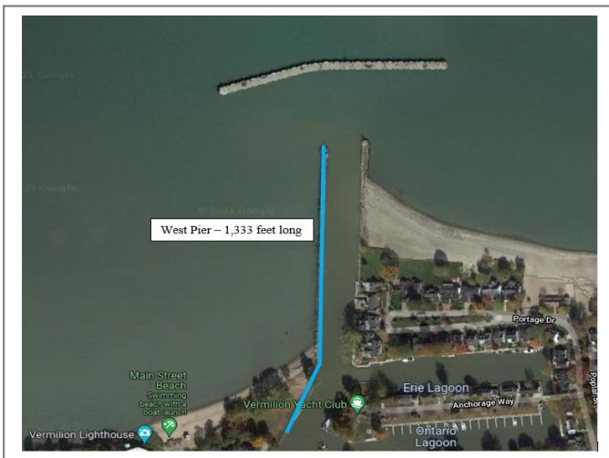
Depicts the entire west pier length
