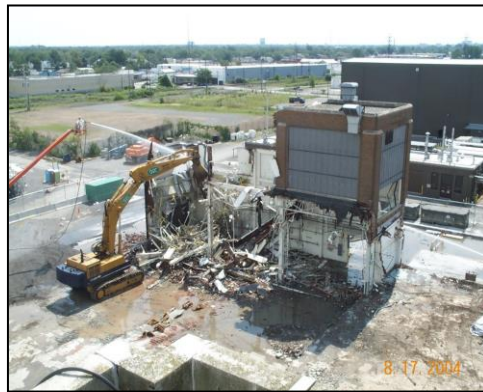
Decommissioning and Demolition
