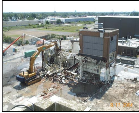
Decommissioning and Demolition
