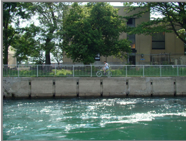
Existing Conditions — Concrete Monolith
