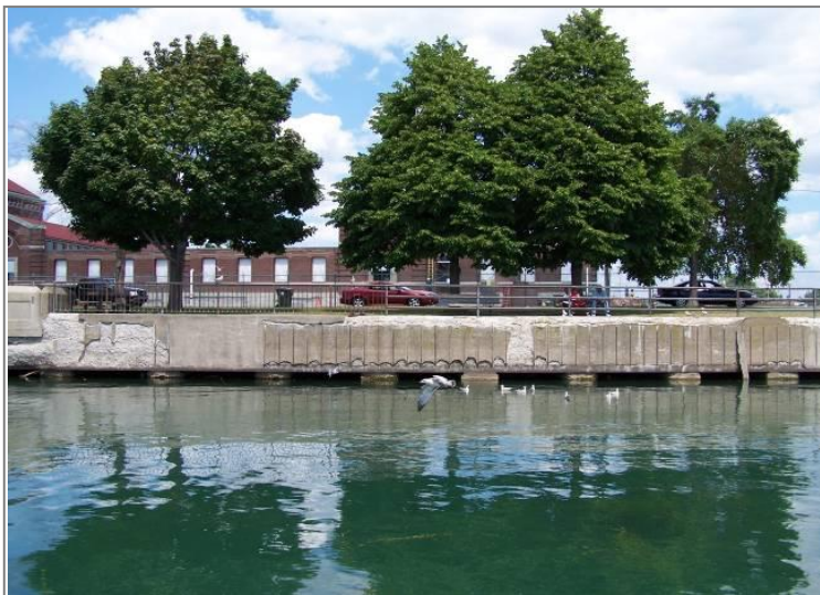
Current Conditions: Concrete Monolith
