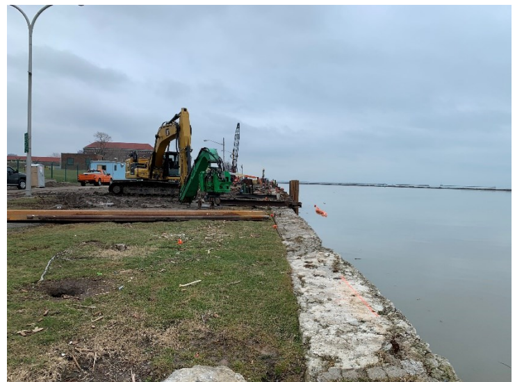
Site under construction January 2021
