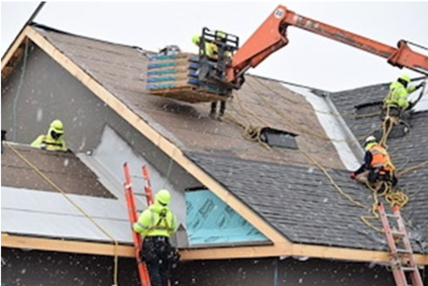
Cottage H/I/J Roofing/Exterior
