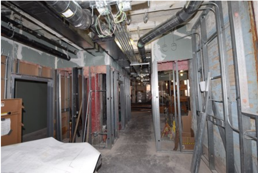
Bldg. 2 Ground Floor Corridor
