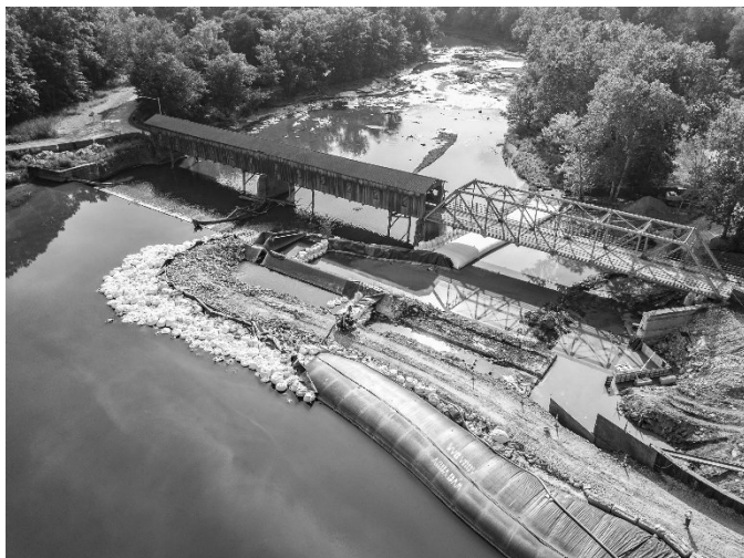
Figure 1: View of the demolition of the existing barrier during construction.
