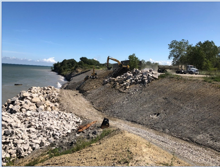
Photo 1 (August 2019) – Access road and early revetment stone staging.
