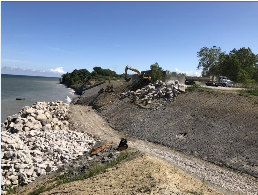
Photo 2 (August 2019) – Access road and early revetment stone staging.
