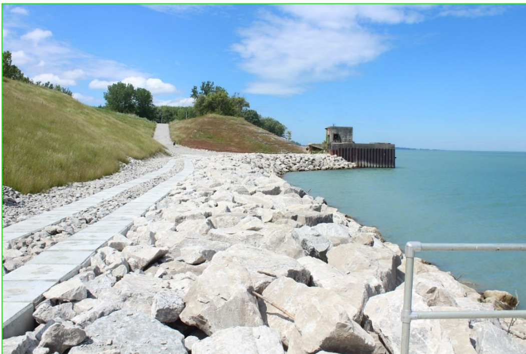
Photo 3 (June 2020) – Completed Revetment
